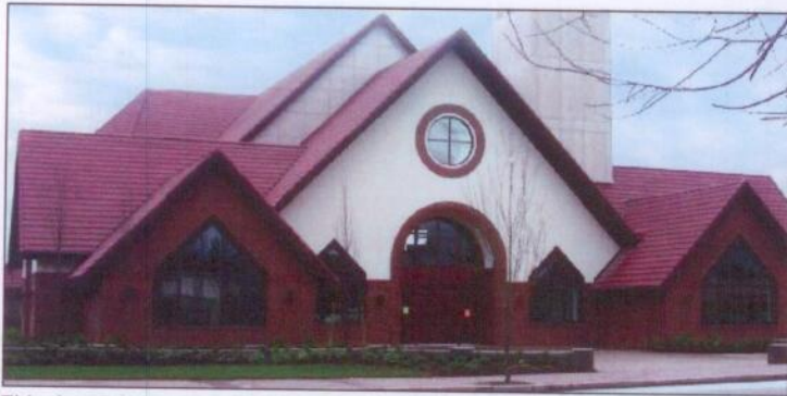
This church in Langley, B.C., made use of tilt-up construction. The top photo shows tilt-up panel exterior walls with exposed glulam wood roof beams. The panels also form part of the interior where the concrete arches were enhanced with a stucco finish to provide a traditional theme. The church's exterior with textured stucco and brick added to enhance the exterior finish of the panels, is pictured on the bottom—proof tilt-up has moved beyond the warehouse.
