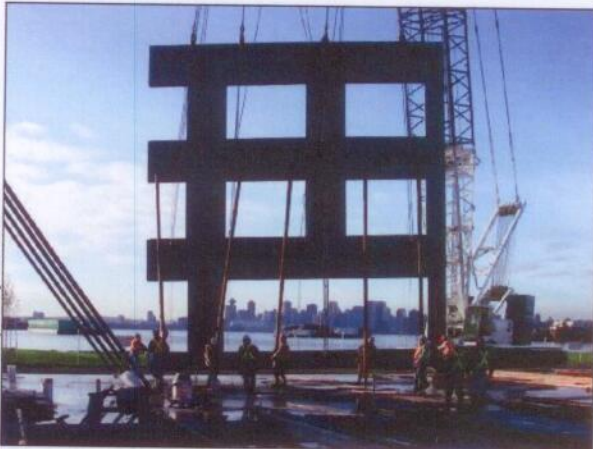
Pictured here is panel for a three-storey office in North Vancouver, overlooking the city skyline. The 9 x 12-m (30 x 40-ft) panel weighs nearly 45,000 kg (100,000 lb).
