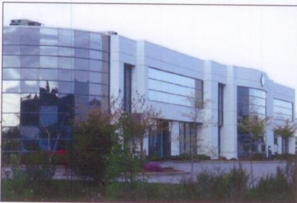
Tilt-up construction was used to build this two-storey office/warehouse building in Coquitlam, B.C.
